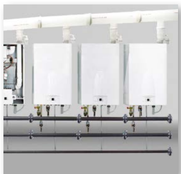
Installation of up to 4 modules in battery
